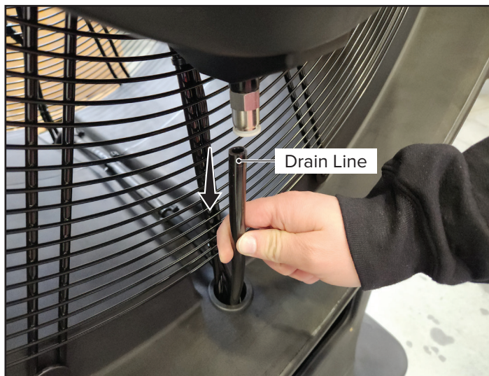
Fig. 2.6 Disconnect and save drain line
